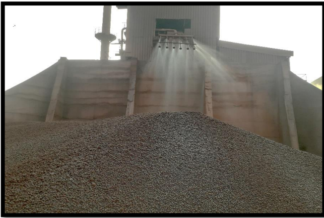
Photographs of water sprinklers installed at yard and pellet transfer point
