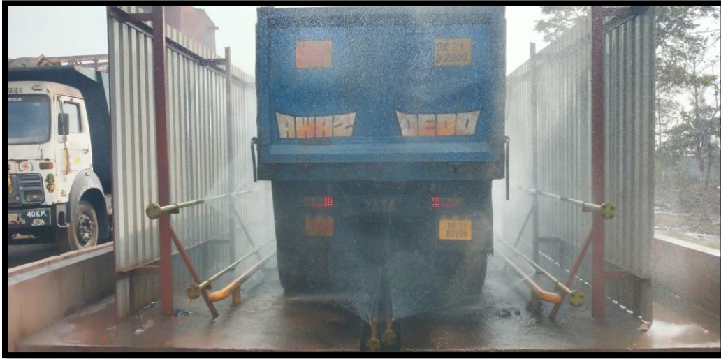
Photograph of Wheel Washing System
