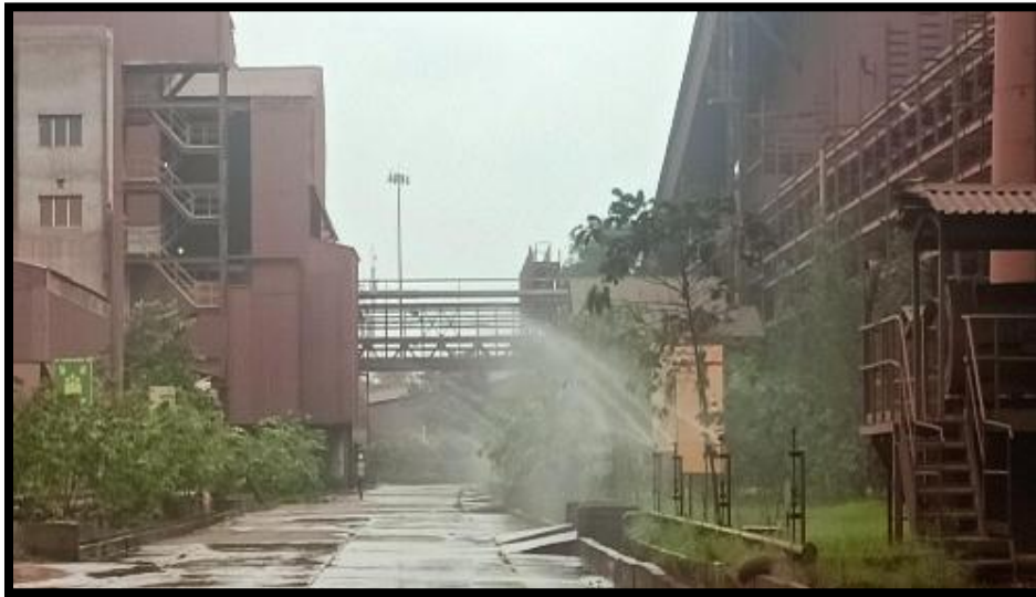
Photographs of fixed water sprinklers on plant road
