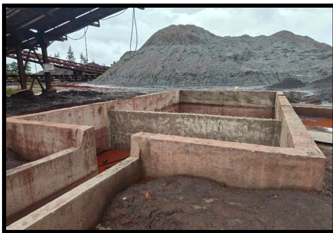
Photographs of settling Pits
