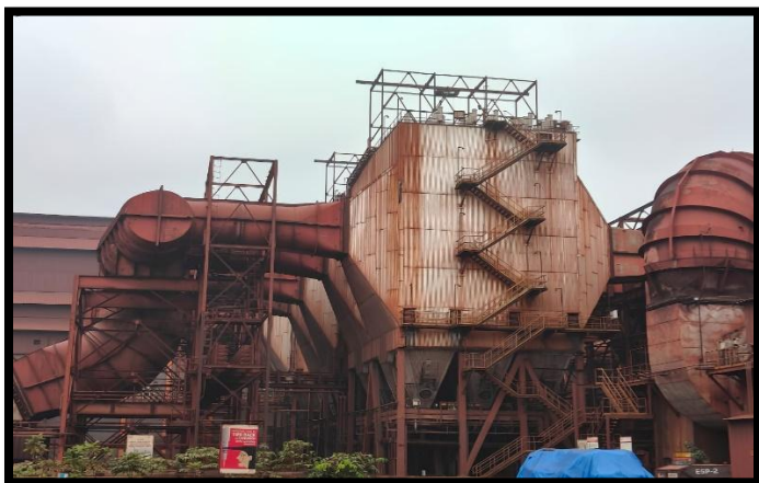
Photographs of Electrostatic precipitator and Wet scrubber installed to capture for Dust generated from process
