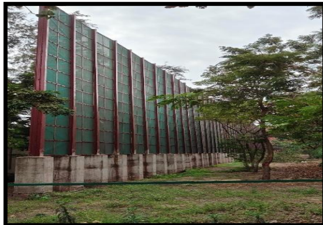
Photograph of Wind screen installed to control fugitive emission towards Musadiha village & IFFCO township
