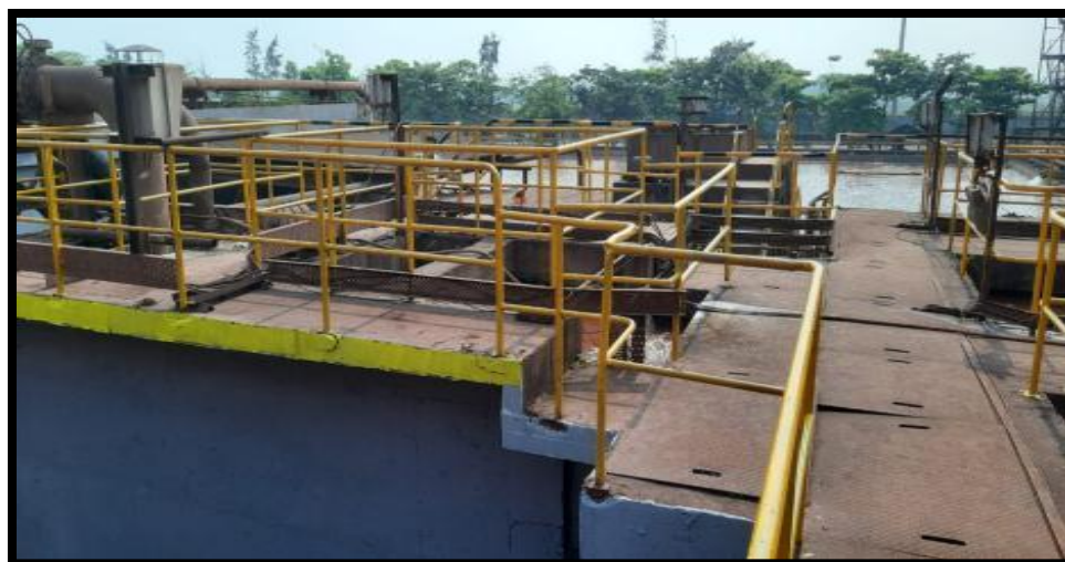
Photograph of installed Water Treatment Plant of capacity 550 m 3 /Hr
