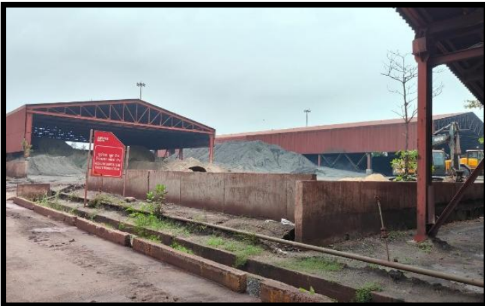
Photographs of toe wall around the raw material yard
